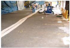
For floors that are not candidates for mechanical or acid etching due to installed equipment, inability to tolerate dust, etc. we offer a special primer called **Flash Bond** that allows our epoxy to stick to virtually any surface, including non porous and sealed surfaces. This is a 1-part product that rolls on fast and easy. Often the cost of this special primer is equal to using mechanical means to prep.
